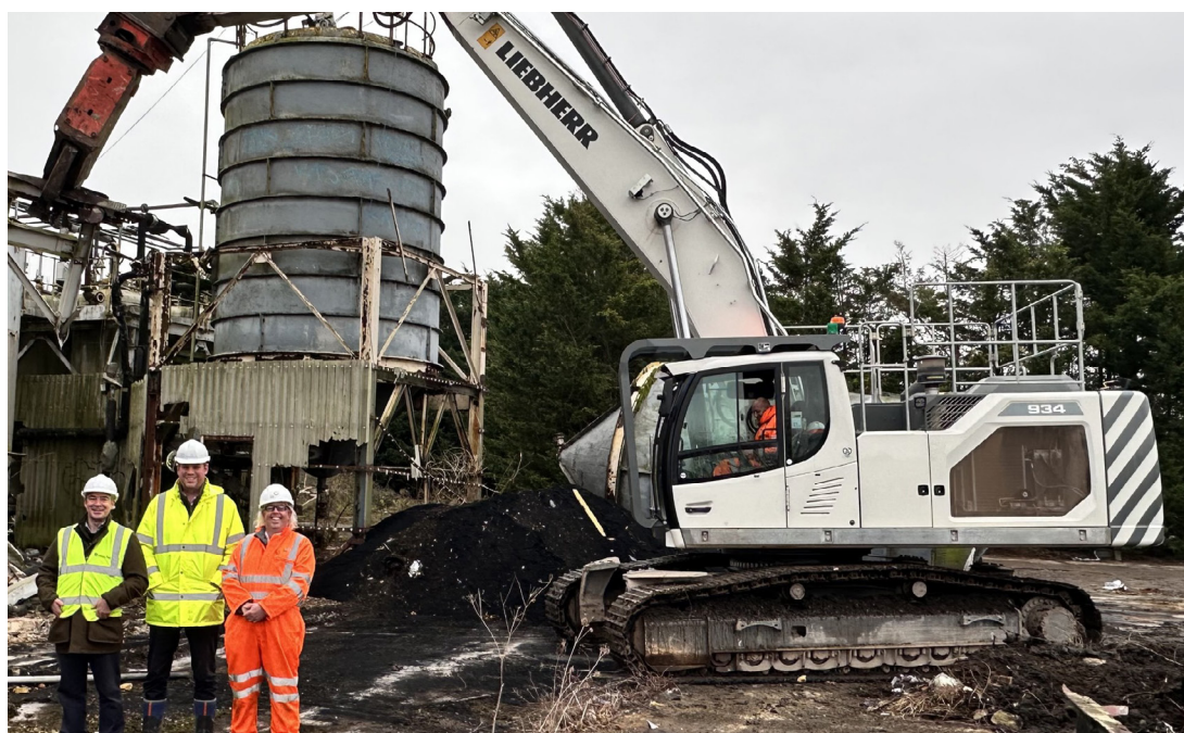
On site at Cambridge Discovery Campus: L to R: Rob Sadler: Foundation Capital Ventures, Simon Green: Bidwells Project Management, Steve Edgar: Vertase FLI.
